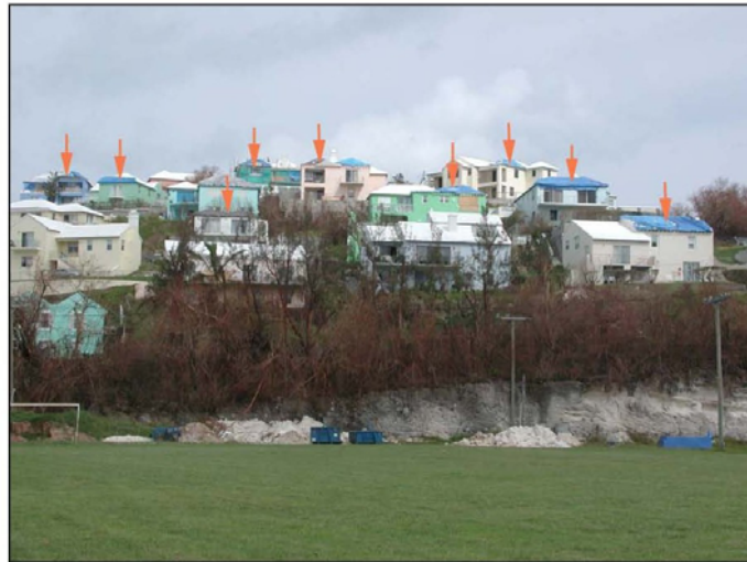
Figure 1. Widespread roof damage on south facing, Loyal Hill, Devonshire.
