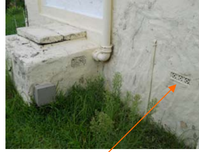
Tank access. Floor vent
