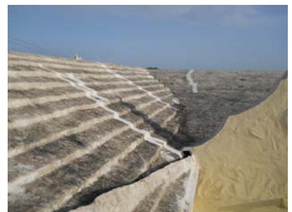
Roof looking north.
