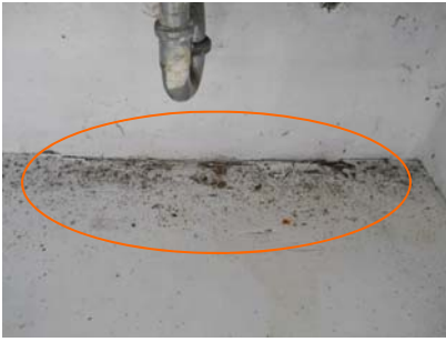
Kitchen base cabinet shows wood rot
