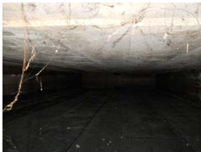
View of inside the tank. Underside of floor slab shown
