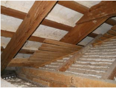
Roof framing is satisfactory
