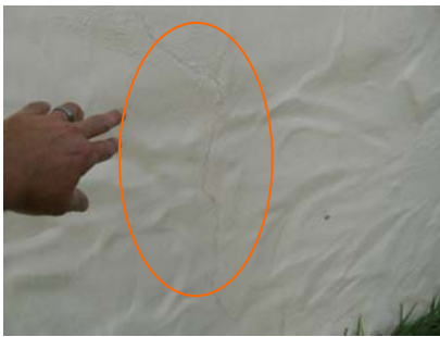
Masonry cracks.
