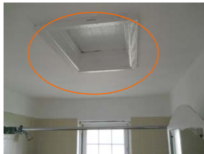
Scuttle hatch in bathroom.
