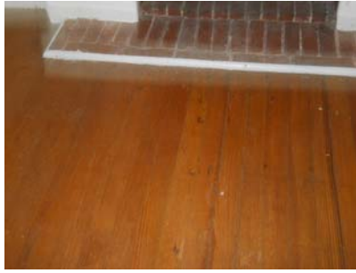
Wood floor at fireplace
