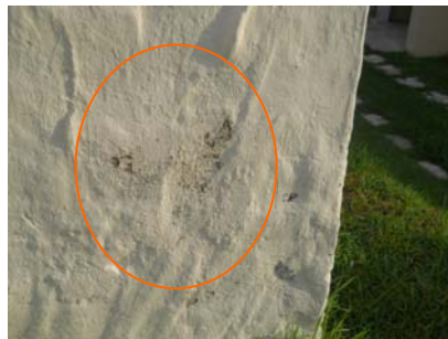
Efflorescence
